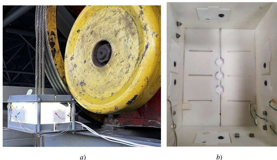
Fig. 3. Hardware component of PAC VIC: a — place in the elevator installation, b — installation points of six IP cameras (the authors' photo)
